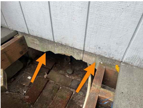
Fiber cement siding (Possible asbestos)
