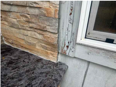
Rotted siding/improper manufactured masonry veneer installation
