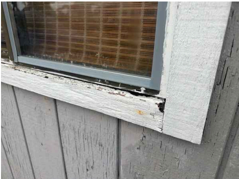
Failed/damaged siding and trim
