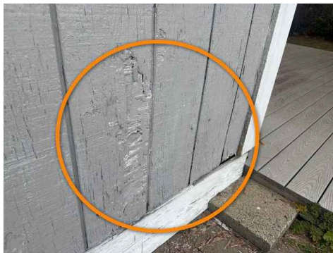
Failed/neglected siding
