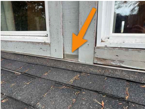
Rotted siding/improper manufactured masonry veneer installation
