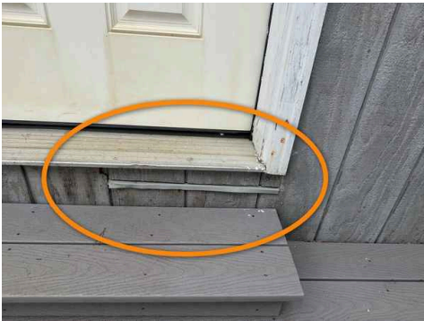
Failed/damaged siding and trim
