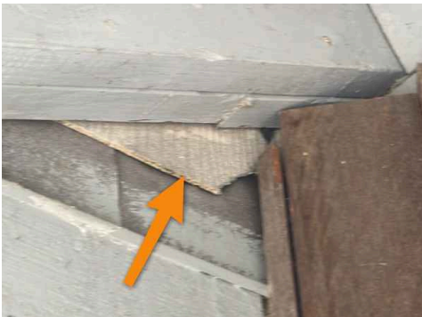
Fiber cement siding (Possible asbestos)
