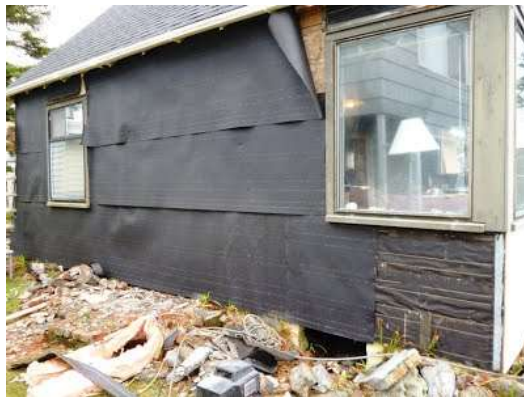
Left: We carefully removed the asbestos shingles and prepared them for transporting to the Hillsboro dump that accepts this sort of waste (for a huge fee). Right: The brick side porch was no longer useful, so it got broken up and removed.
