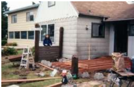
Left: Mick installed decking for the wind screen. Right: We installed floor joist on 12" centers. The deck is built of Trex, a product made from plastic and sawdust. Trex isn't as sturdy as real wood, so we needed lots of joists to support it firmly.
