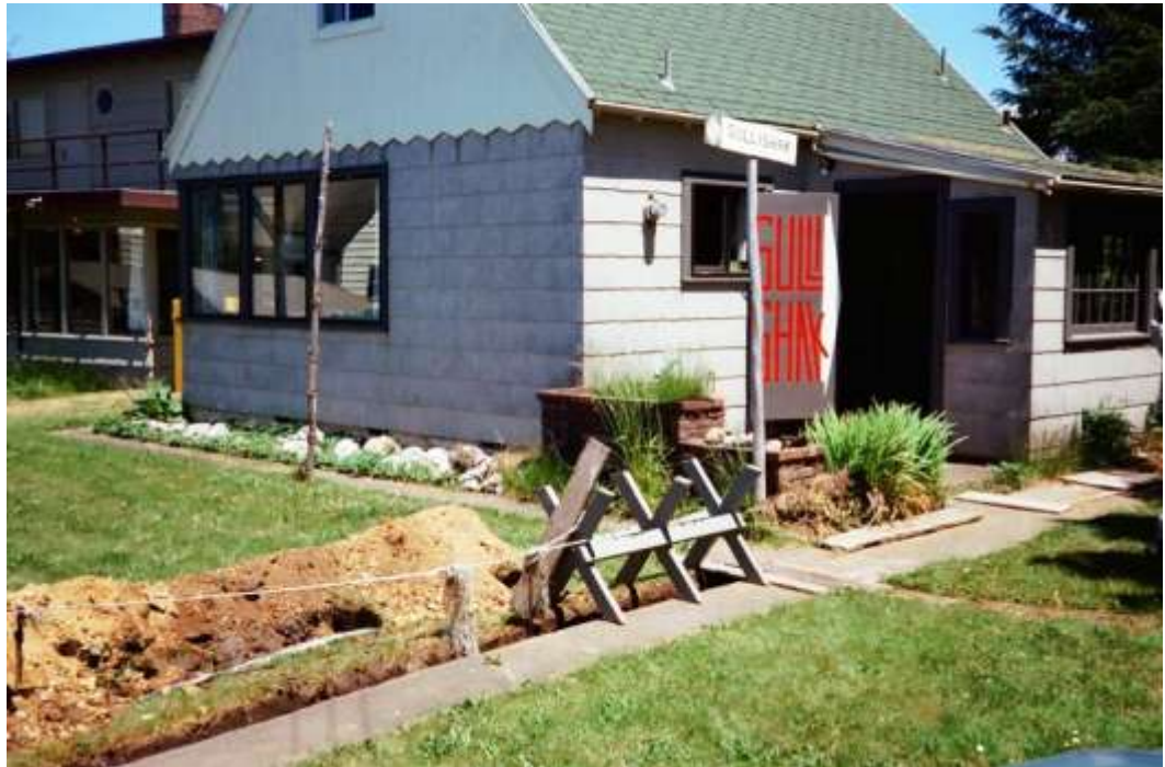
Putting in the sewer line in 1976.
