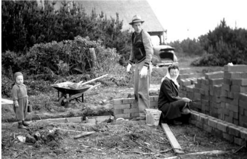
Wes, Elsie and Steve lay the foundation blocks for Sullishak. Nancy is in the car's back seat. Note that Wes and Elsie are mixing the mortar by hand.
