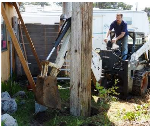
Left: Chris Reiter used his Bobcat to lift the large telephone poles in place to support the new deck.
