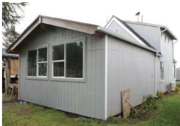
The exterior is now finished on the new family room.
