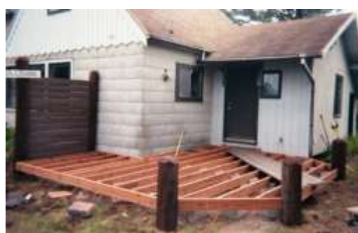
Left: Mick installed decking for the wind screen. Right: We installed floor joist on 12" centers. The deck is built of Trex, a product made from plastic and sawdust. Trex isn't as sturdy as real wood, so we needed lots of joists to support it firmly.
