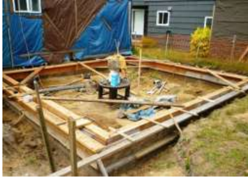
Left: Work began with building concrete forms from scrap lumber.
