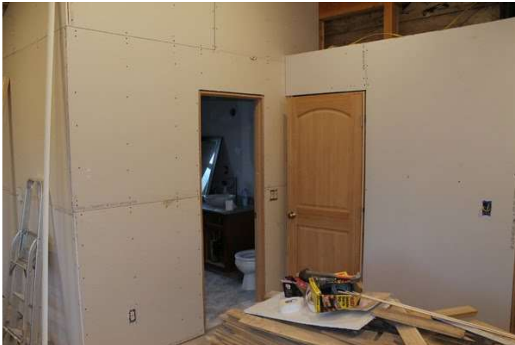
Here we are in the new family room looking back at the door to the main cabin. On the left is a new bathroom with tile floor.
