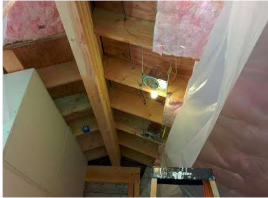
Left: We added lights and insulation to the new family room.
