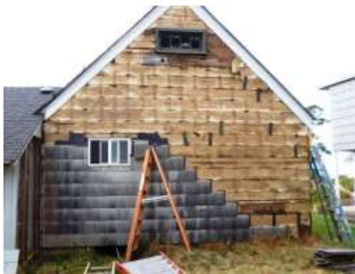
Left: We carefully removed the asbestos shingles and prepared them for transporting to the Hillsboro dump that accepts this sort of waste (for a huge fee). Right: The brick side porch was no longer useful, so it got broken up and removed.
