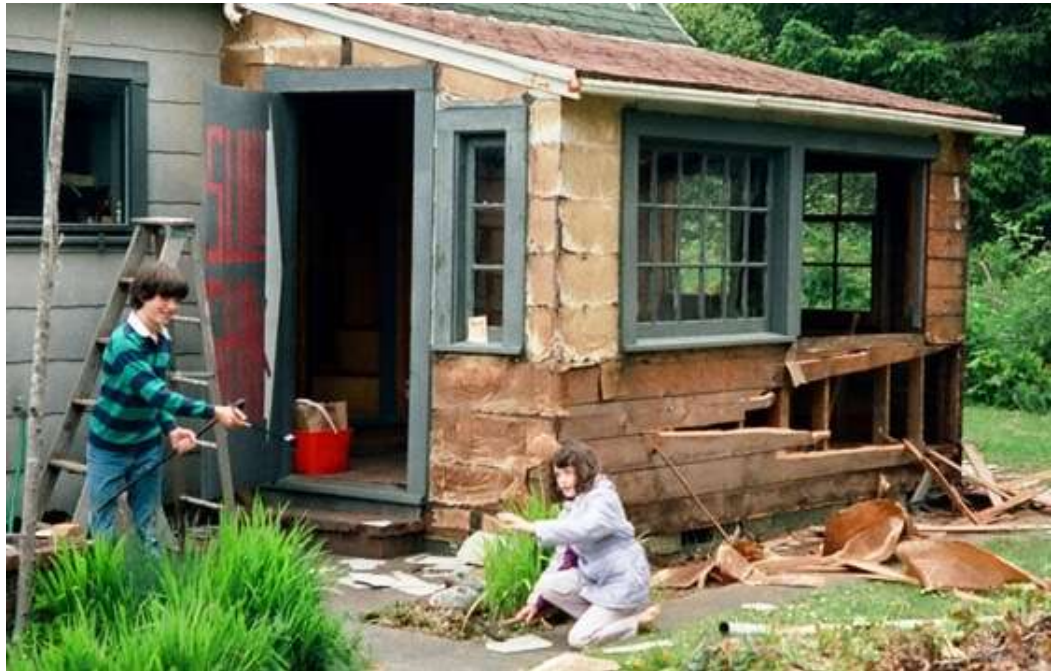
Joel Sullivan and Gail Sullivan help tear down the rotten side porch.
