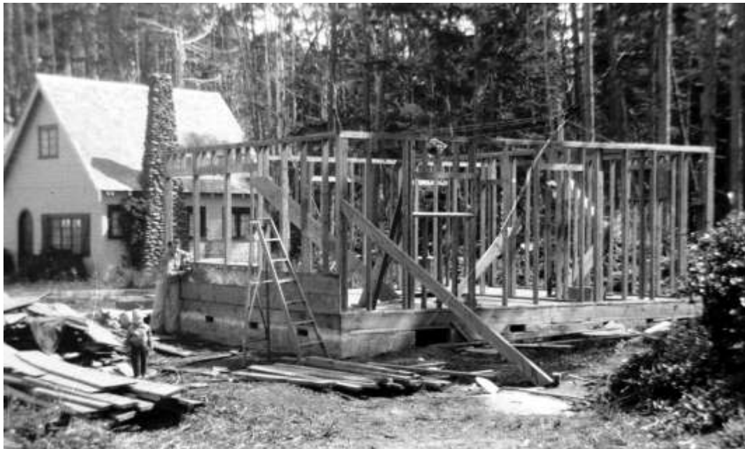
Elsie and Steve at Sullishak as the walls go up in the summer of 1947.
