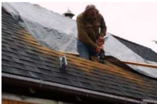
Left: Dave Sullivan used a Sawzall to cut into the roof to create new upstairs dormers.
