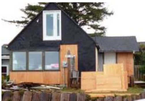
Left: New siding went up in front. Right: A deck was suspended temporarily on 4-by-4s.
