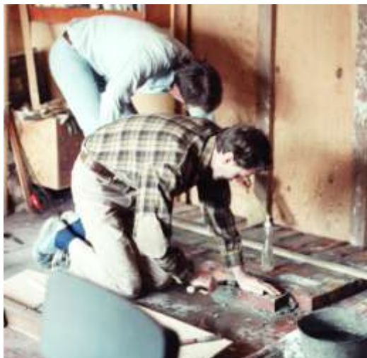
Dave and Steve begin laying bricks for the wood stove.
