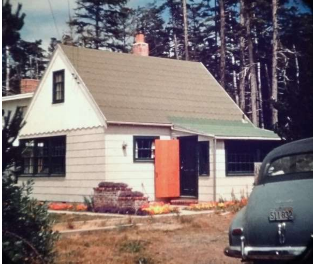
The sun porch has been finished, sidewalks have been installed, and Orma Sullivan paid a mason to construct a planter at the front of the patio.
