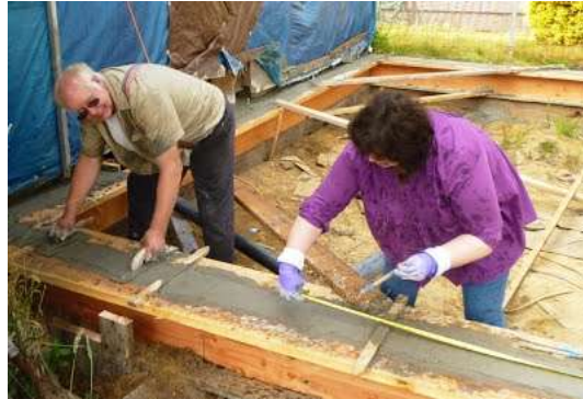
Left: Work began with building concrete forms from scrap lumber.
