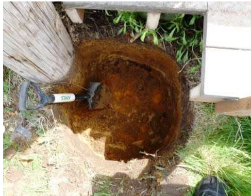
Left: To support the new deck, we dug footings.
