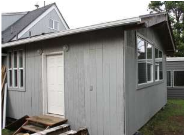
This view of the back of the cabin is where a storage shed has been replaced by a new family room.
