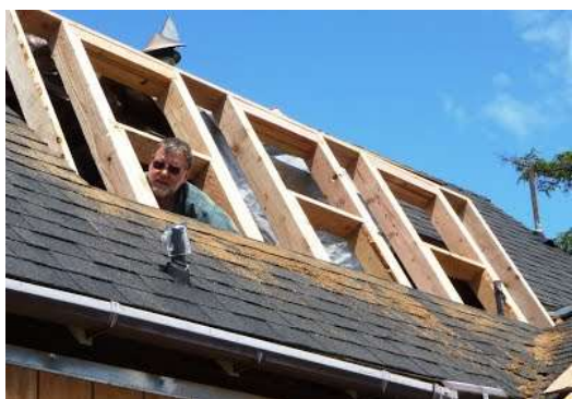
Left: Bob Woodworth raised a wall for the new dormer.
