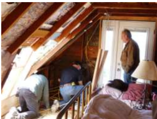
Left: Dave Sullivan used a Sawzall to cut into the roof to create new upstairs dormers.
