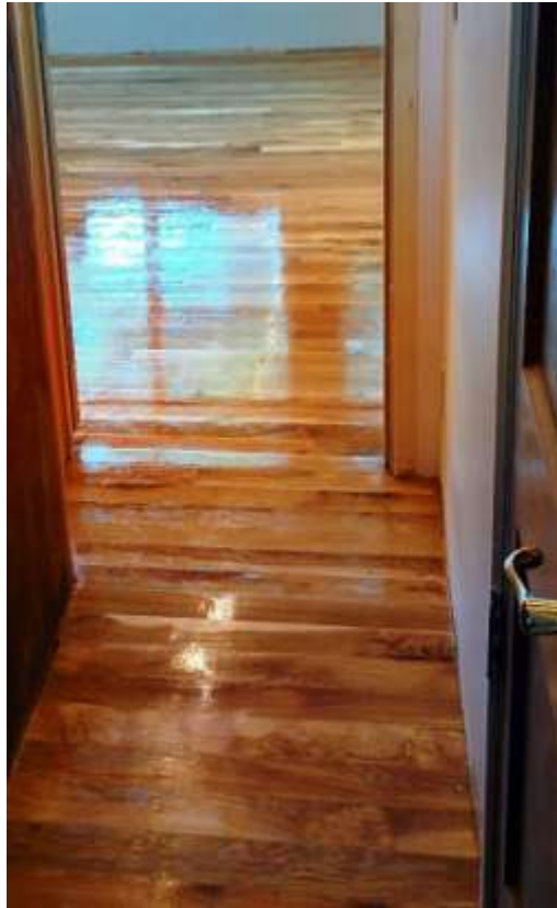
Left: The transition from the family room to the original cabin came out better than we expected. Because we built the new family room about 1-1/2 inches too low, you have to walk uphill to get into the new cabin.
