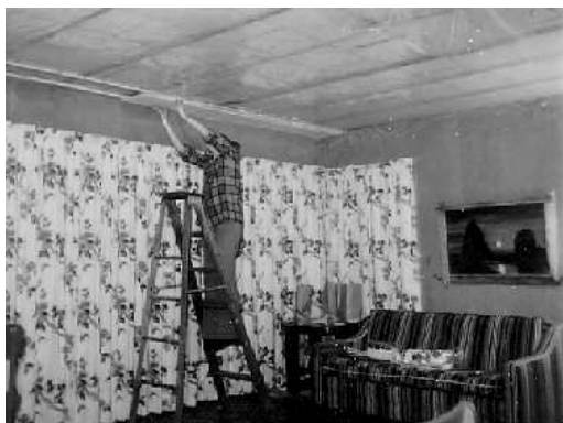
Then, Janet installs ceiling tiles.
