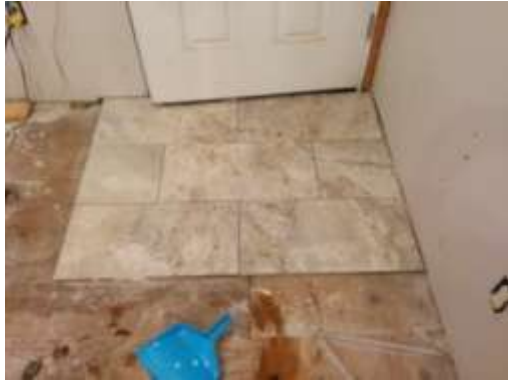
Left: We added drywall and a tile entryway to the new family room.
