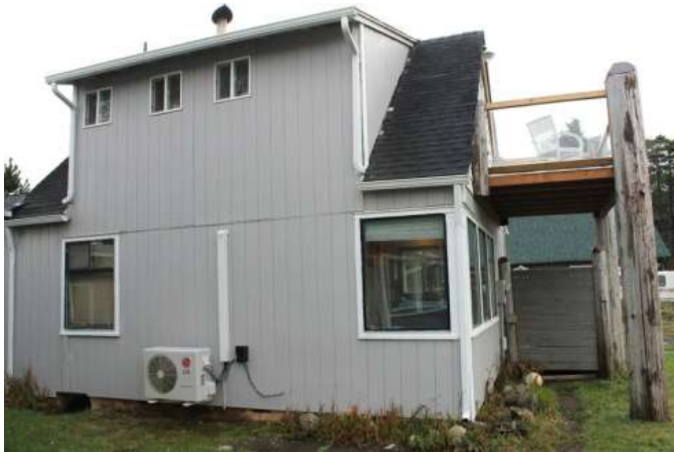
This is north side of the cabin. The new balcony is at the right. The north door and porch that were never used are gone. Note the outside unit of a heat pump which provides efficient heat for the living room.
