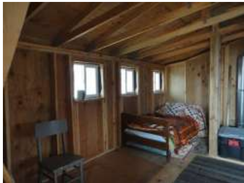
Left: North wall upstairs has been pushed out and roof lifted.
