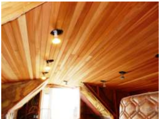
Left and right: The second floor dormers get a new cedar ceiling.
