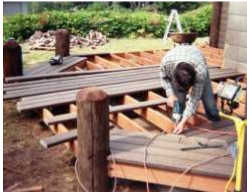
Left: Bill attaches a piece of Trex with a wood screw. We used Phillips head screws, and they weren't easy to install because the bit kept popping out of the slots.
