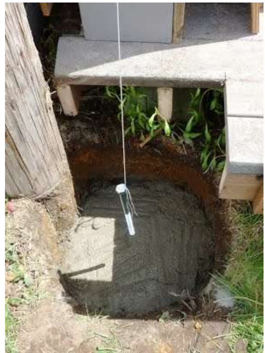
Right: Although it wasn't structurally necessary, we poured concrete in the bottom of the footings.
