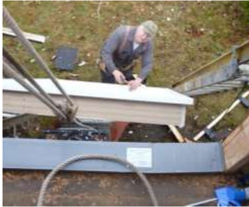
Left: Dave Helton steadies the new second-story door as it gets raised with a block and tackle. Right: The door looked silly at first: it lead to a 12-foot drop-off.
