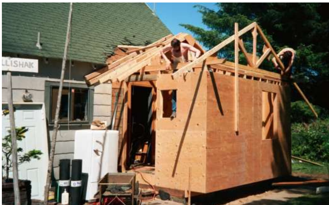
Dave and Bill Sullivan install rafters for the replacement porch.
