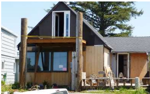
Left: Chris Reiter used his Bobcat to lift the large telephone poles in place to support the new deck.
