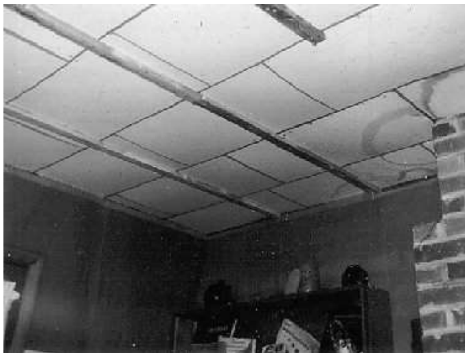
The second picture in the series shows furring strips running across the tiles.
