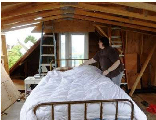
Right: The new scissor trusses have been installed, so Barb Sullivan made a bed in the unfinished upstairs.
