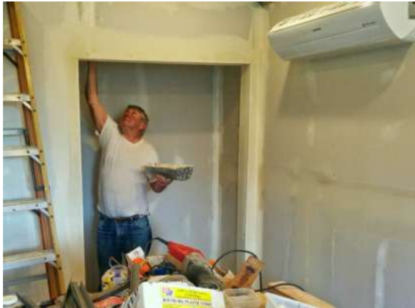
Gary Anderson applied the drywall mud and tape to the new addition.
