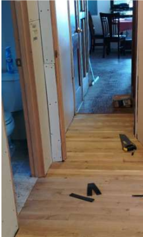
Left: The transition from the family room to the original cabin came out better than we expected. Because we built the new family room about 1-1/2 inches too low, you have to walk uphill to get into the new cabin.
