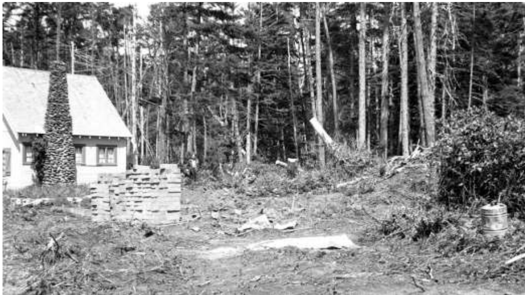
Concrete blocks for the Sullishak foundation have been delivered, and the Sullishak site has been cleared by a bull dozer leaving large piles of brush to the side and rear. Vera Lantz is just barely visible looking back at the camera from her home site's location.
