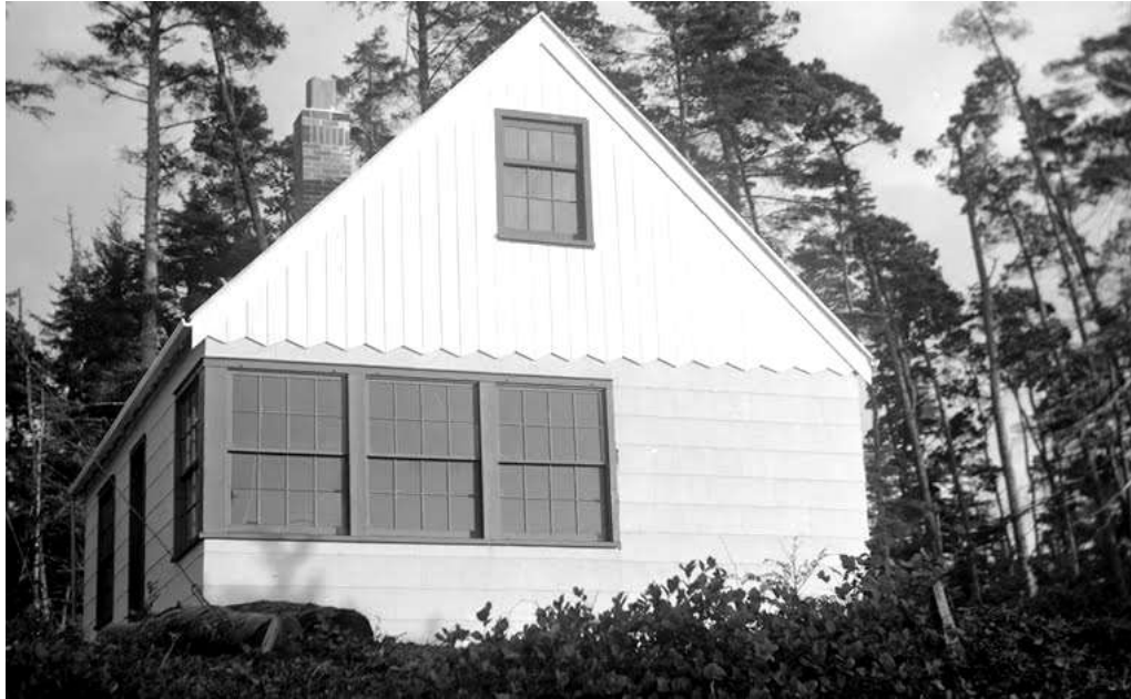
The finished cabin with asbestos siding.
