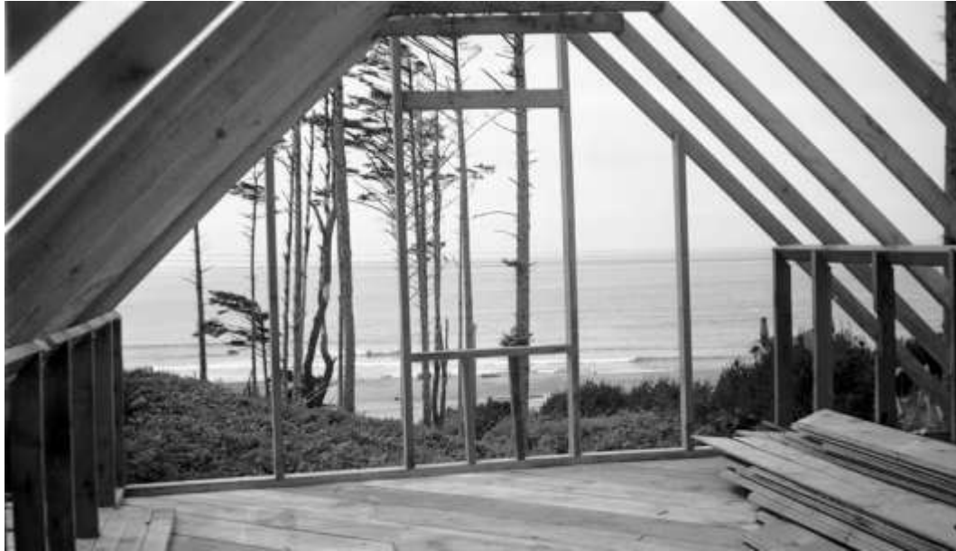
Notice how the subfloor runs diagonally across the cabin.
