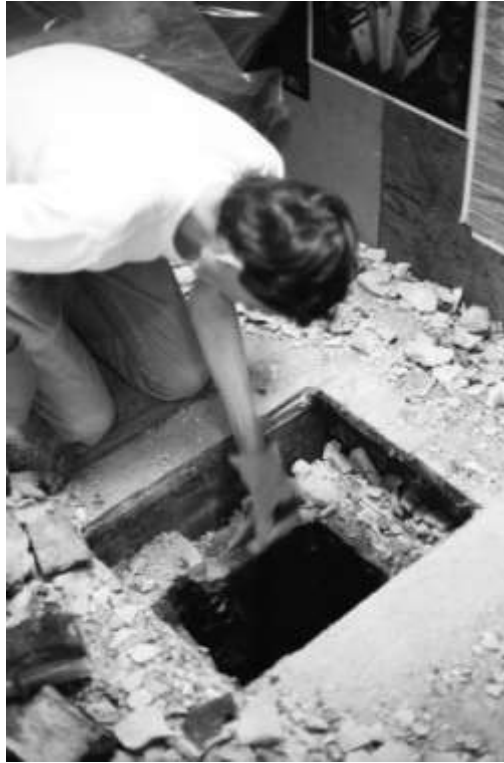
Steve attempts to remove chimney bricks in the first-floor's ceiling.
