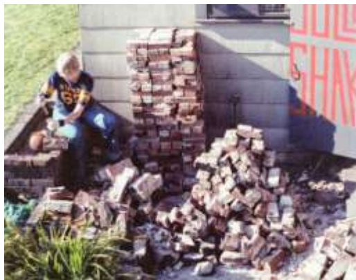
Janet Schmidt cleaned most of the brick.
