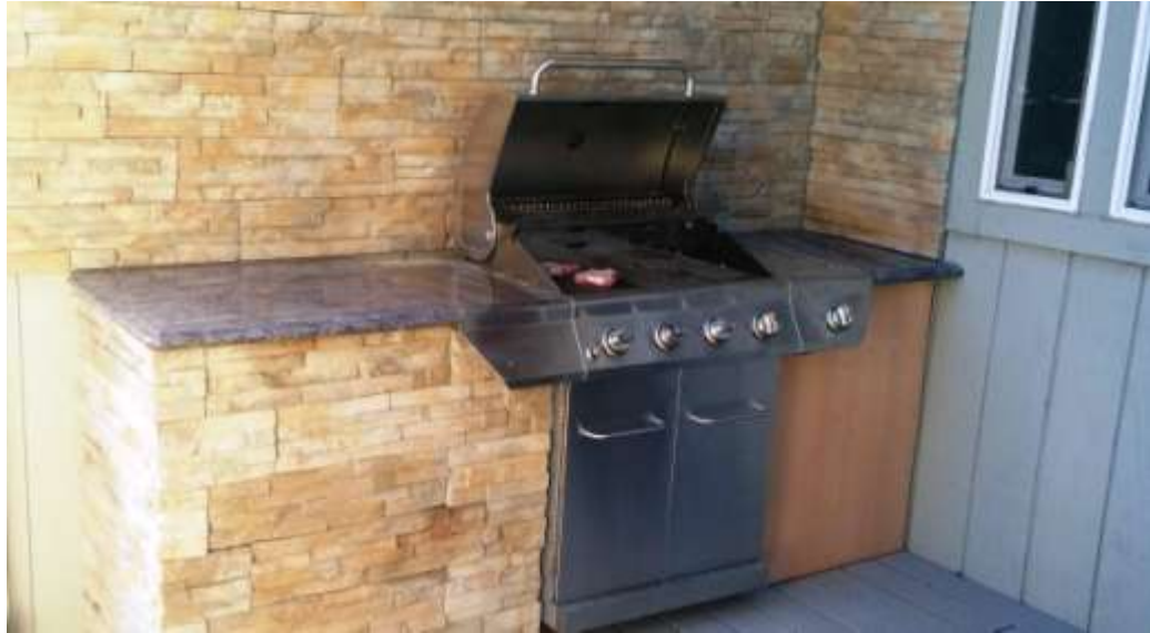
The almost completely installed grill gets its first assignment: a pair of pork chops.
