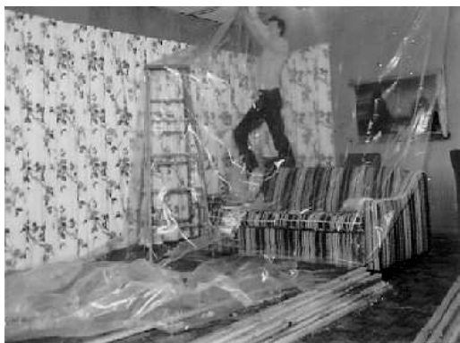
Next, Dave puts up plastic sheeting.
