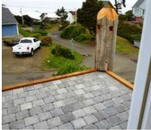
Left: The new deck got a layer of pavers.
