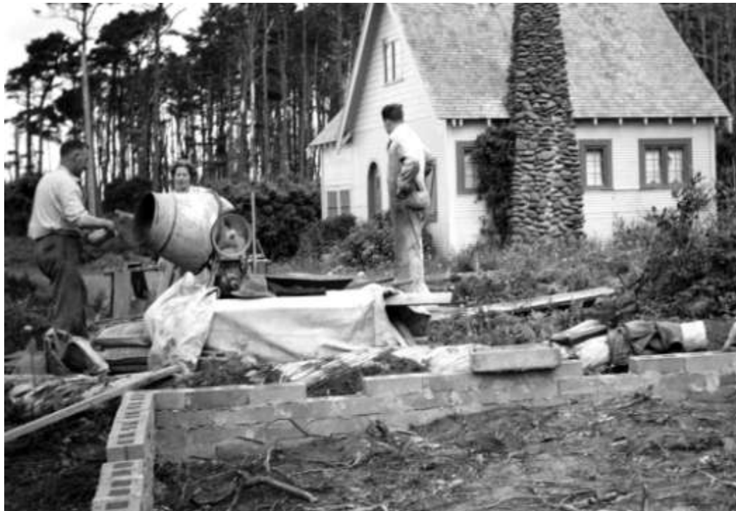
Vera and Jewell Lantz (and some unknown helper) begin building their home next door. They use an electric mixer for their foundation.
