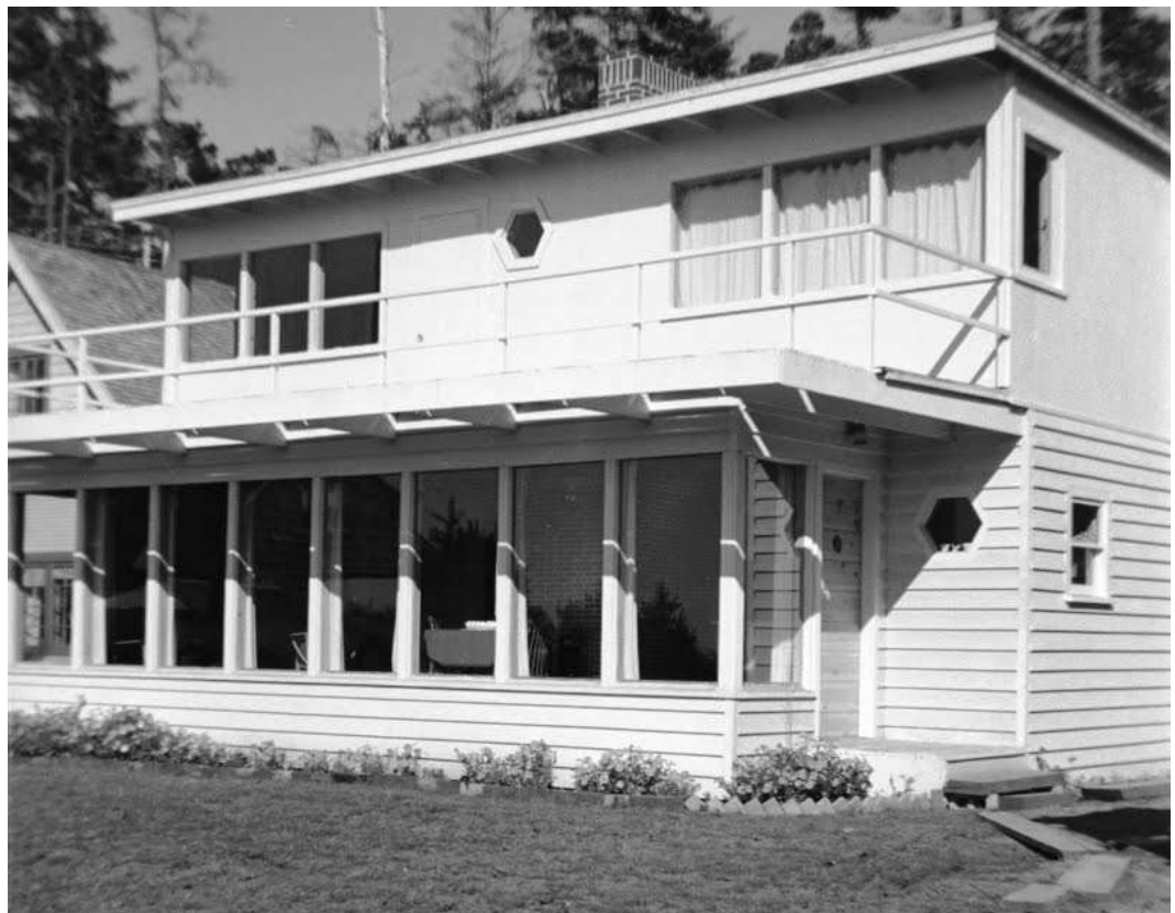
The Lantz home (which is just north of Sullishak) shortly after its construction was completed. Note the use of wood planks as a sidewalk.
