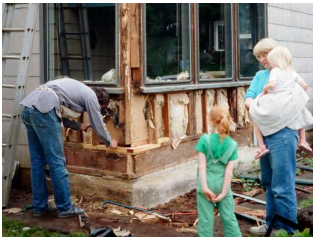
Dave repairs rotten walls below the front windows while Mary, Molly and Janet watch.
