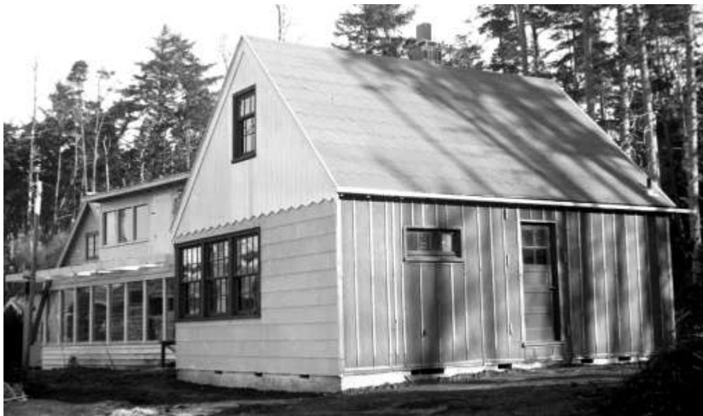
The cabin at the end of the 1947 construction season: The south side is covered with tar paper.
