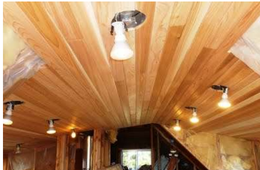
Left and right: The second floor dormers get a new cedar ceiling.
