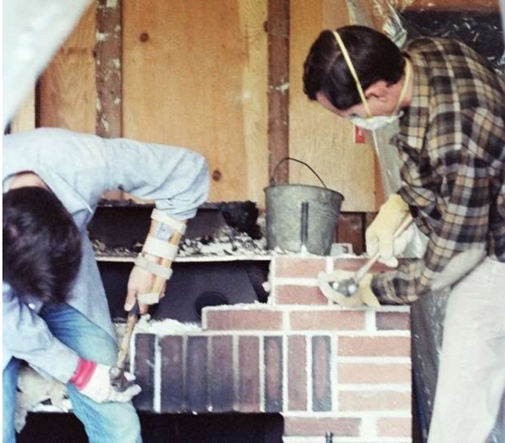
Dave and Steve remove the brick fireplace.
