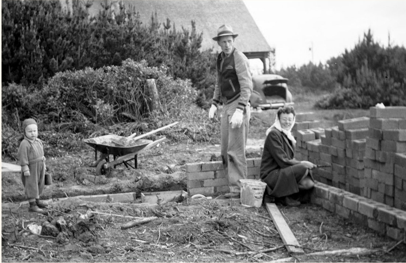
Spring 1947. Wes and Elsie Sullivan lay the foundation blocks, mixing the mortar by hand, while Steve, who was three, plays beside them. Two-month-old Nancy is asleep on the back seat of the 1940 Mercury.
